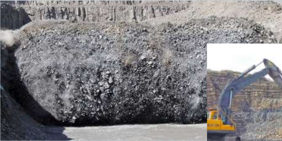
Blasting creates fines
